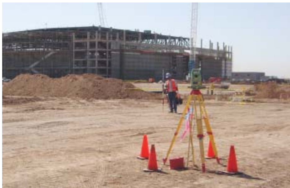
ASAM surveyors used the Leica SR530 GPS receivers and many TPS 1100 and 1103+ Professional Series robotic total stations from their inventory for the critical staking needed to complete the project.
